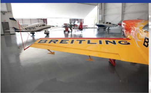
When it comes to protecting the floors of airplane hangars, there is much to consider. The flooring system must be slip and impact resistant, able to withstand heavy loads and resistant to hazardous chemicals.
